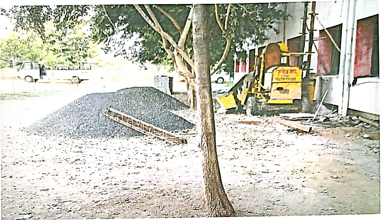
4.4.2 Maintenance Work (a)
